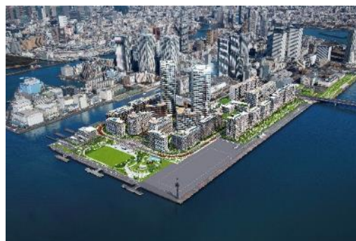
CG illustration of completed exterior
