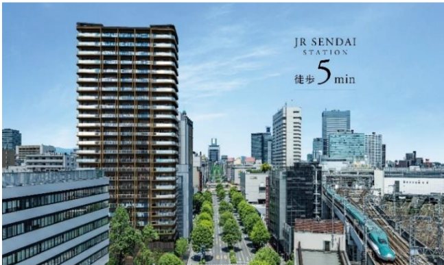
【CG illustration of completed exterior】
