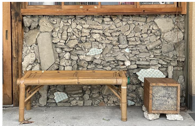
Stone wall utilizing of concrete waste (reference)
