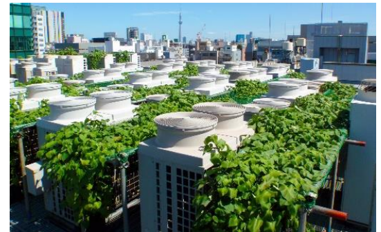
Rooftop system for planting sweet potatoes around external air conditioning units (image) Source: Sumitomo Corporation
