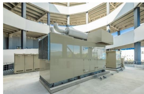
Emergency generators for 72 hours of power
