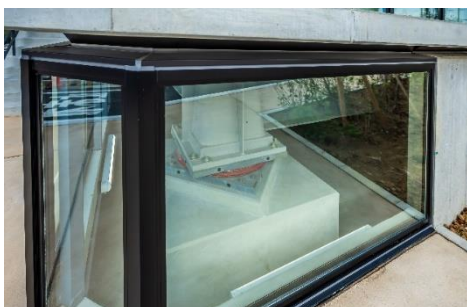
Seismic isolation system
