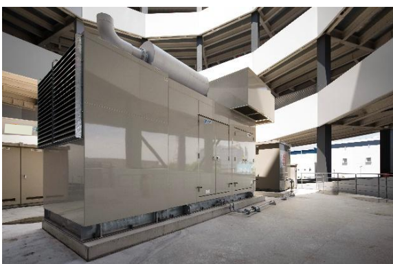
Rendering of emergency power generator
