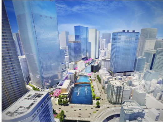
Bridge after removal of the Metropolitan Expressway viaduct*
