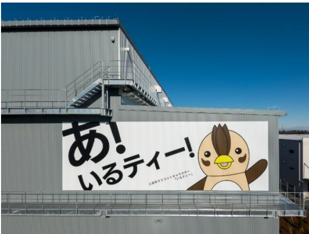
Promotional sign (on the south-facing wall of the building)
