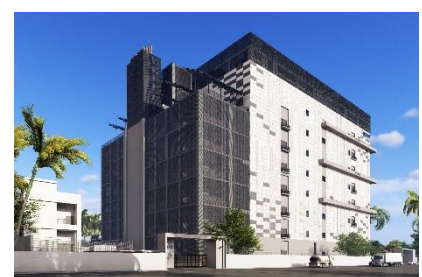
CapitaLand Data Centre, Chennai 01
