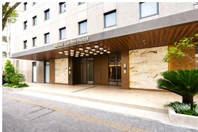
Mitsui Garden Hotel Okayama entrance exterior
