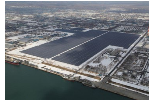
Tomakomai Solar Power Plant
