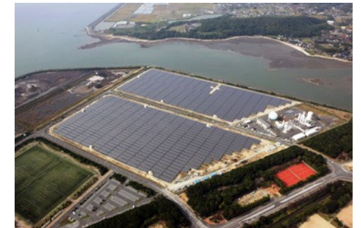
Hachinohe Solar Power Plant
